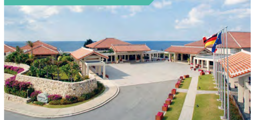
Bankoku Shinryokan Resort MICE Facility
