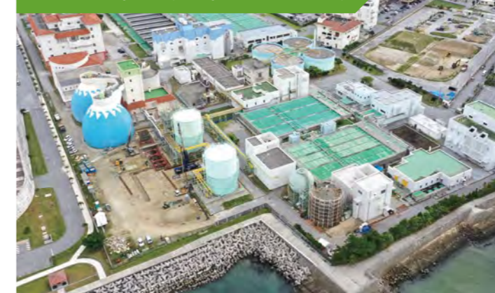
Naha Sewage Treatment Center cleans up sewage
