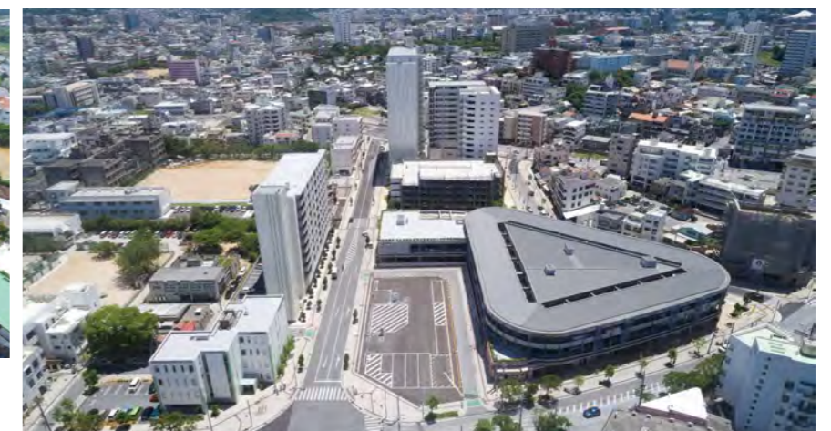
Naha Nouren zone was modified to improve its function as a disaster prevention block
