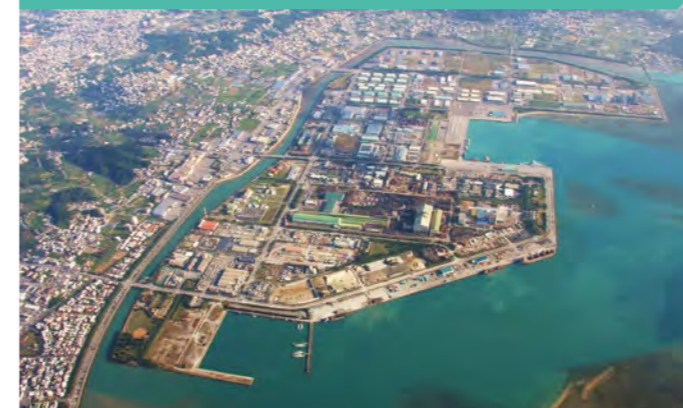
Nagagusuku Port is being developed to bolster industry (New Port Zone)
