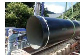
Water supply facility renovation planned and earthquake resistance promoted
