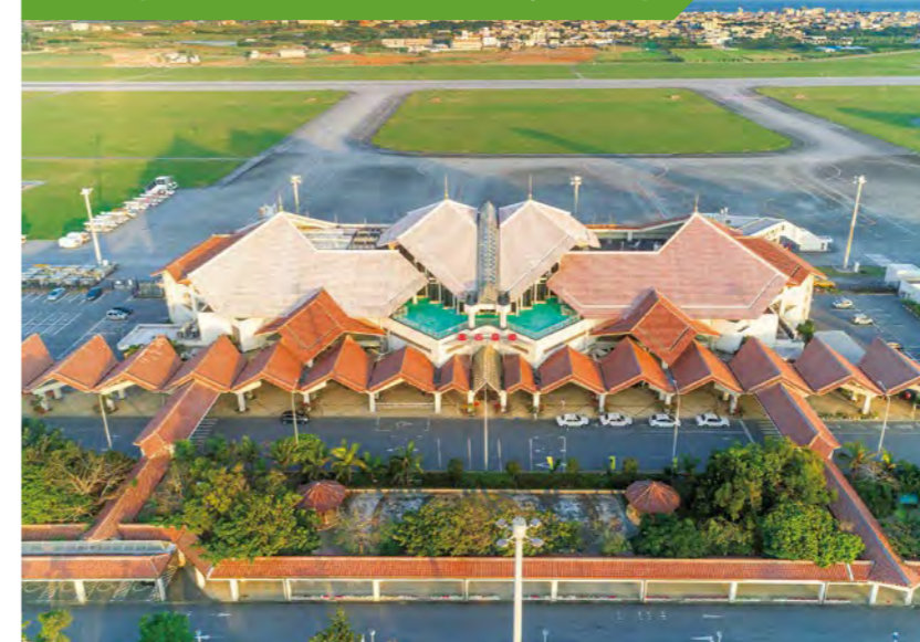
Miyako Air Terminal building designed based on the motif of the city's official bird the grey-faced buzzard
