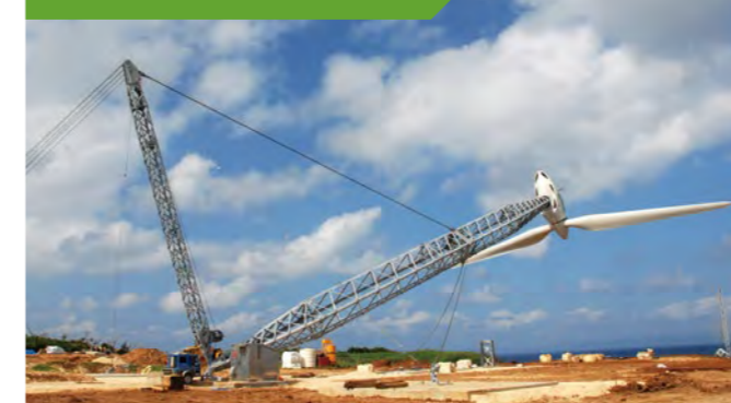
Retractable wind turbines that fold over during typhoons Courtesy of The Okinawa Electric Power Company, Incorporated
