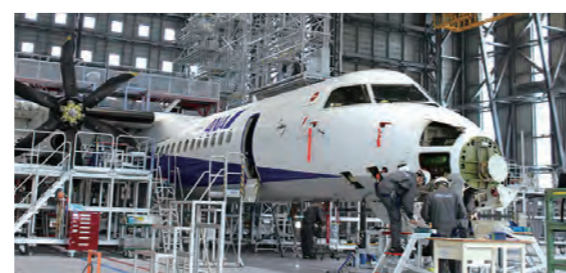
Maintenance of aircraft (Large dock inside the aircraft maintenance facility, MRO Japan Co., Ltd.)
