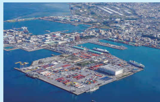
Naha Port International Container Terminal P.12~
